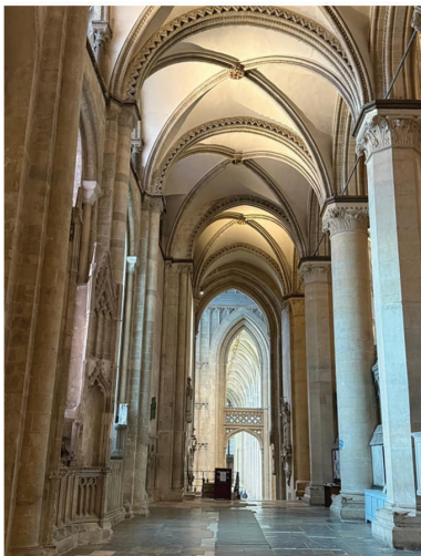
Prime example of Gothic architecture, featuring distinct pointed arches and ribbed vaults
